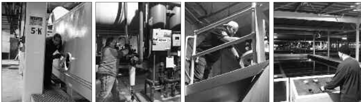
Local 399 members at the Jardine Water Purification Plant (left to right) Ramon Lopez inspecting traveling screens, Michael Schifano switching Instrument Air Dryers, Chris Browne checking low lift pump for vibration and Barry Ecklund manually backwashing filter.
