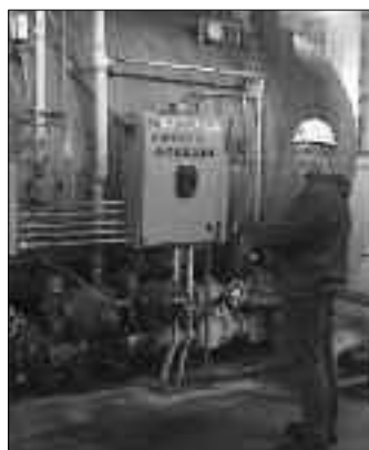
Local 399 members at the Metropolitan Water Reclamation District (left to right) George Mangan checking a Babcock and Wilcox water tube boiler in the central boiler facility. John Yanahan checking the sludge screens in the concentration building. Eric Brummel checking the boiler in the digester. John McNamara filling the water softener brine tank.
